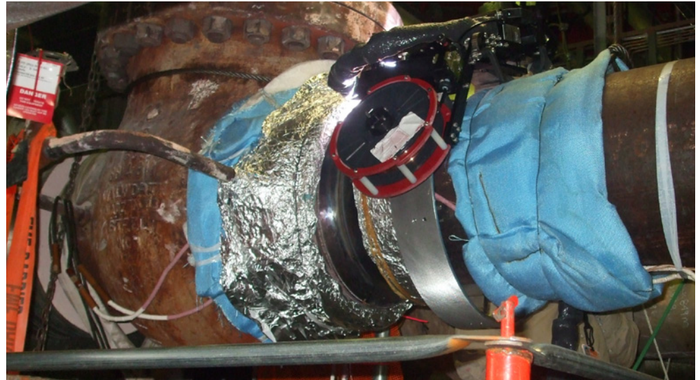
Above: These beautiful uniform rows of filler metal reflect excellence in pre-programmed, auto-positioned bead placement and illustrate the precise distance between the weld paths. Below: The downhill travel of the DualARC™ orbital weld head shows the wire spool and the mounting track placement.
