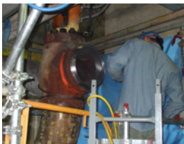
Above: The precision 37° bevel with "J" land prior to welding.
