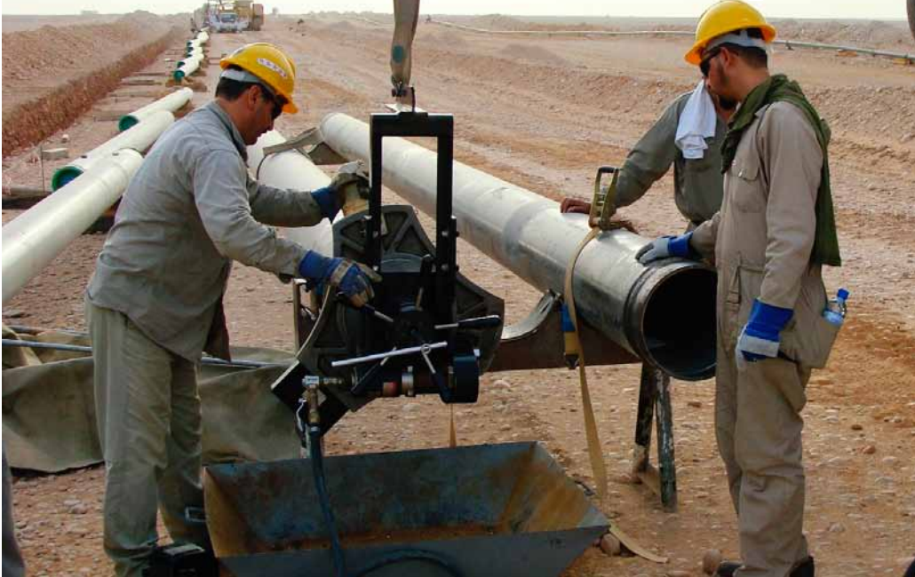
The classic Model 224B in a non-classic role as the primary weld prep tool for a special land-based pipeline with Inconel lined bore.
